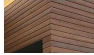
ACCENT PANELS ORANGE METAL PANEL CEDAR SHIPLAP
